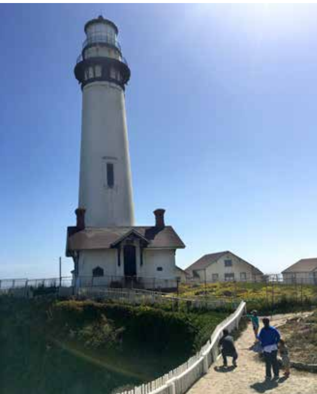
Lighthouse and attached oil house.
