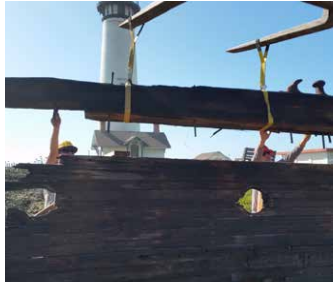
Installation of the hull of the Point Arena Schooner that shipwrecked at the modern-day Park in 1913.
