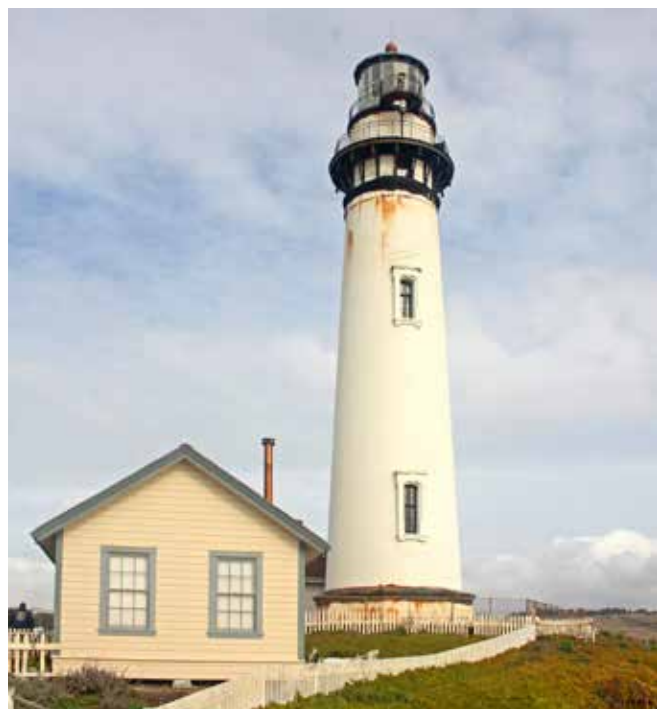
View of Lighthouse and Carpenters Shop from overlook behind the Fog Signal Building.
