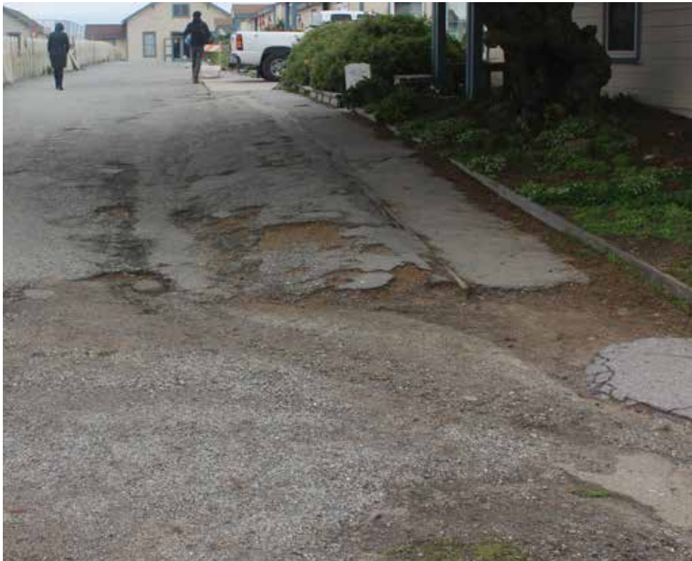
Uneven paving along main pathway in the Light Station
