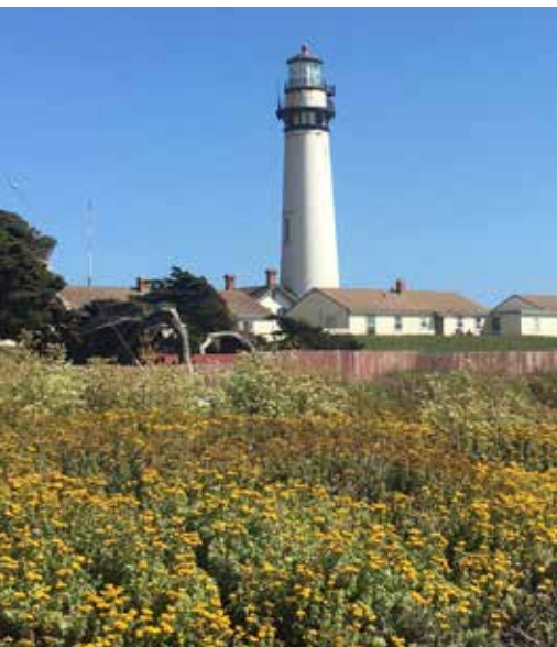
The Lighthouse is an important historic cultural resource in the Light Station.
